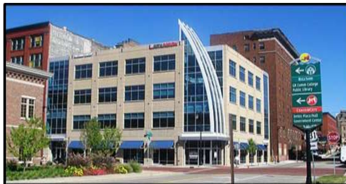
Figure 2 - Grid 70 Building next to 35 Oakes Street
